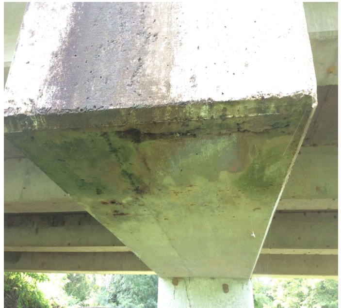
PHOTO 2 Description The Lt and Rt ends of Bent 5 cap has delaminated areas and spalls with exposed reinforcing steel.
