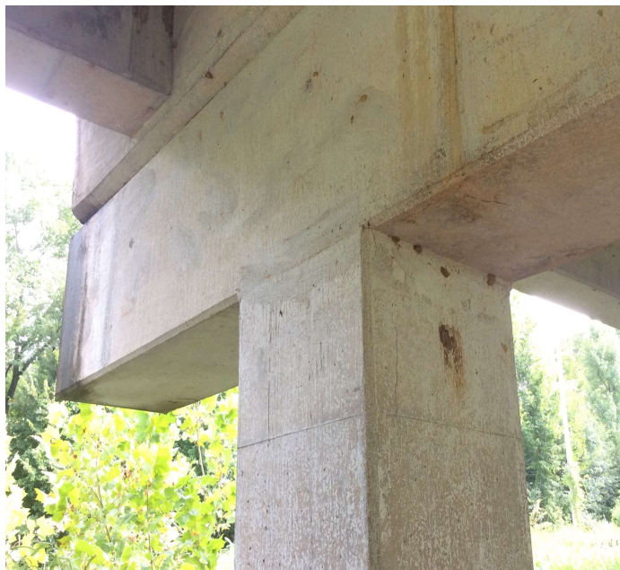
PHOTO 3 Description The Lt and Rt ends of Bent 4 cap has delaminated areas and spalls with no exposed reinforcing steel.
