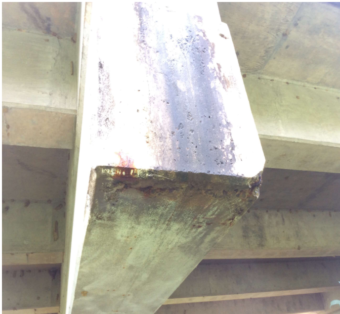
PHOTO 1 Description The Lt and Rt ends of Bent 2 cap has delaminated areas and spalls with exposed reinforcing steel.
