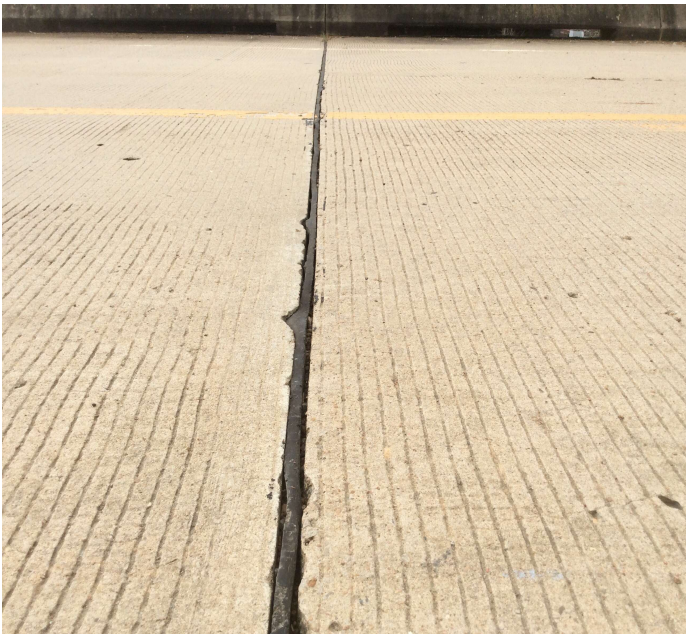
PHOTO 1 Description The deck joints have adhesion failure and appear to leak water.
